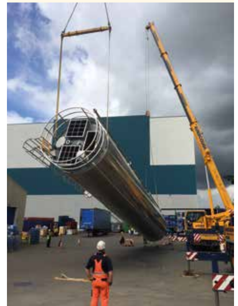
The sugar dissolver silo is installed.
